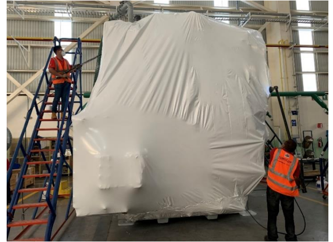
Application of shrink line thermo coating
