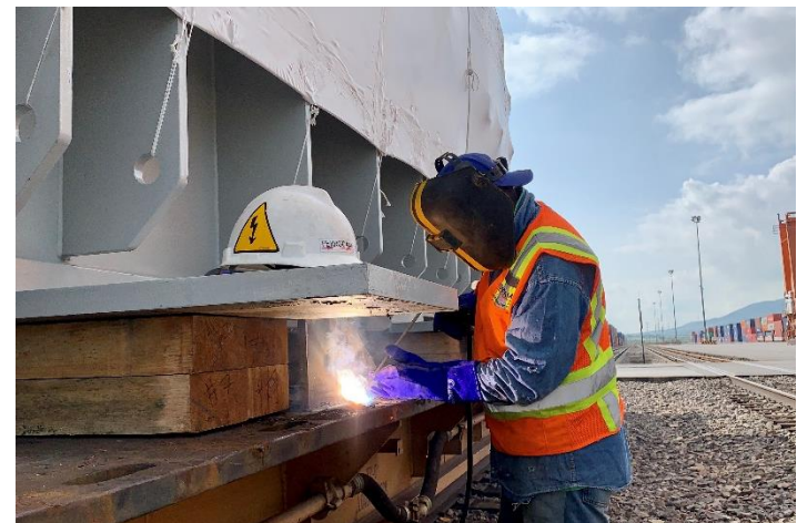
Fixing equipment to platform
